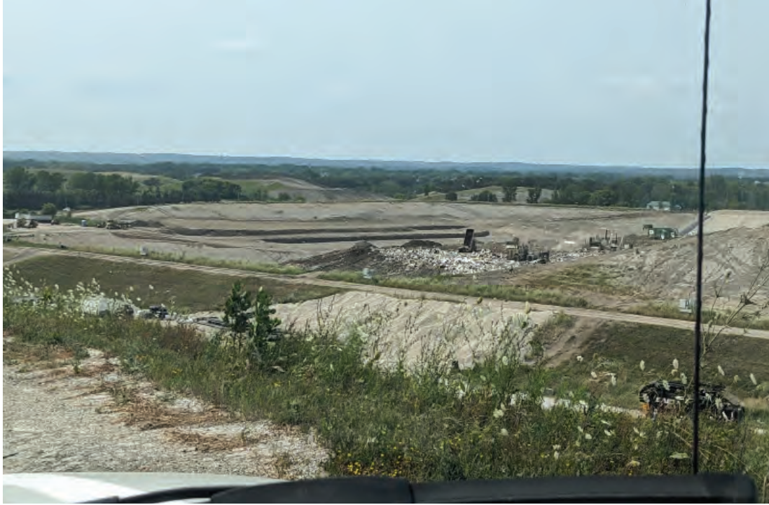
Terraced excavation of future cell
