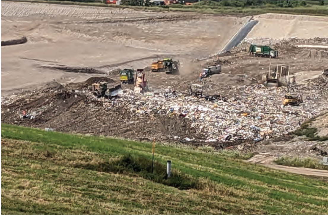
Tipper outside of working face in Phase 3
