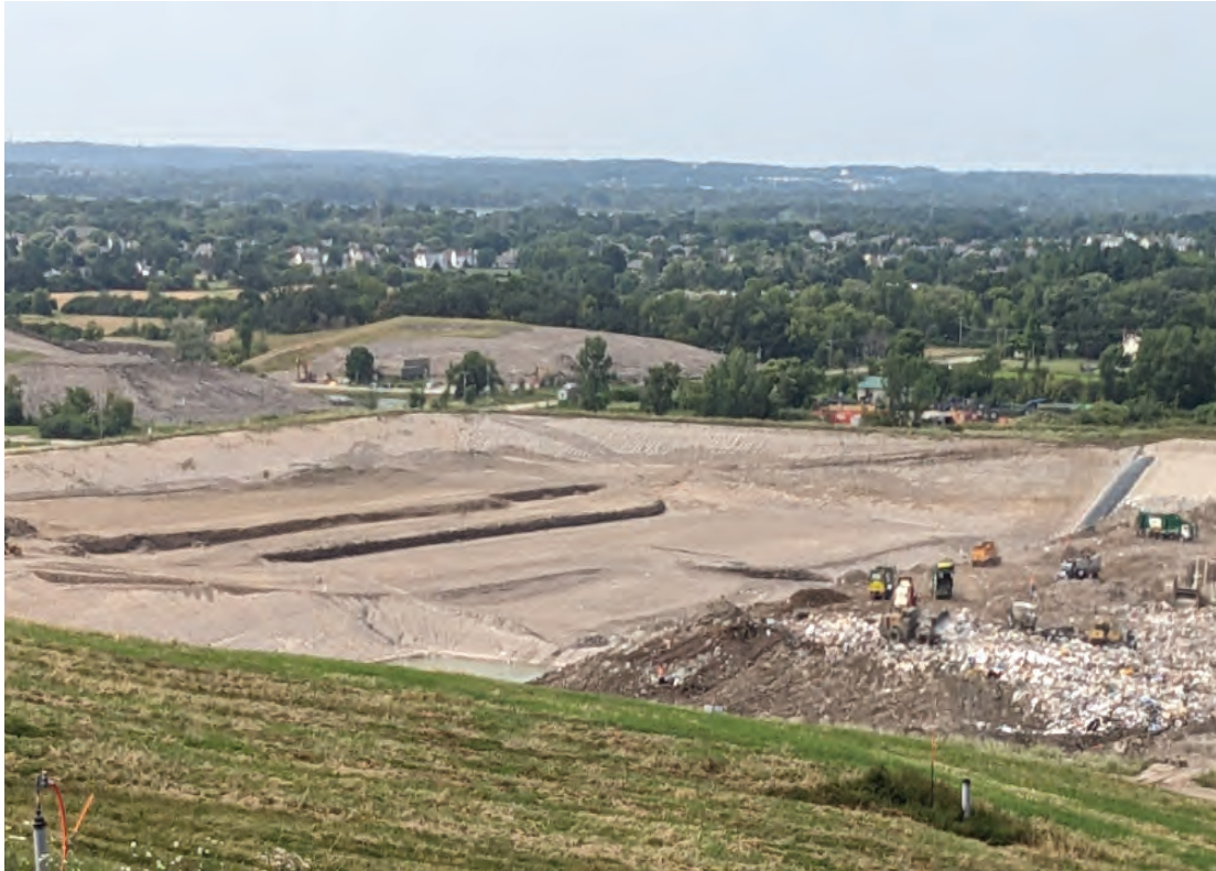
Future cell excavation
