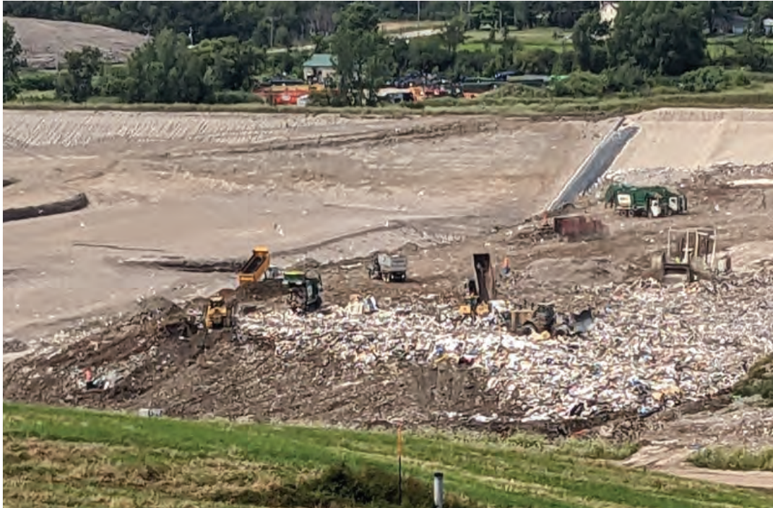
Working face with cover prepared on South edge
