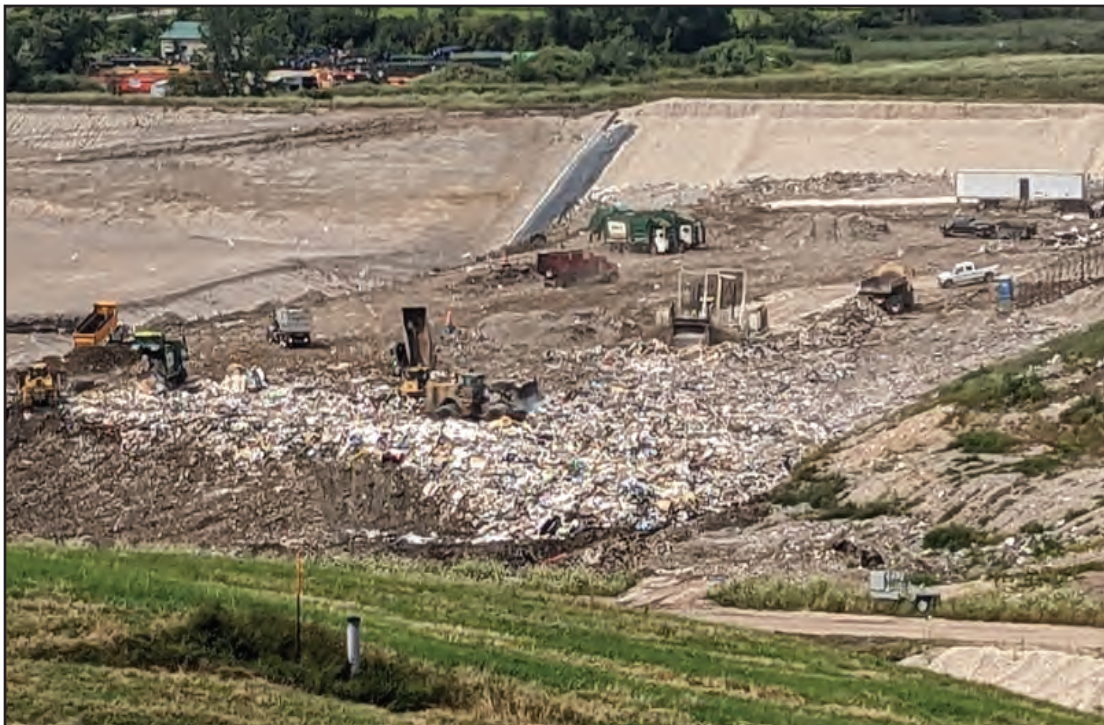
"L" shaped working face in Southeast corner of Phase 3
