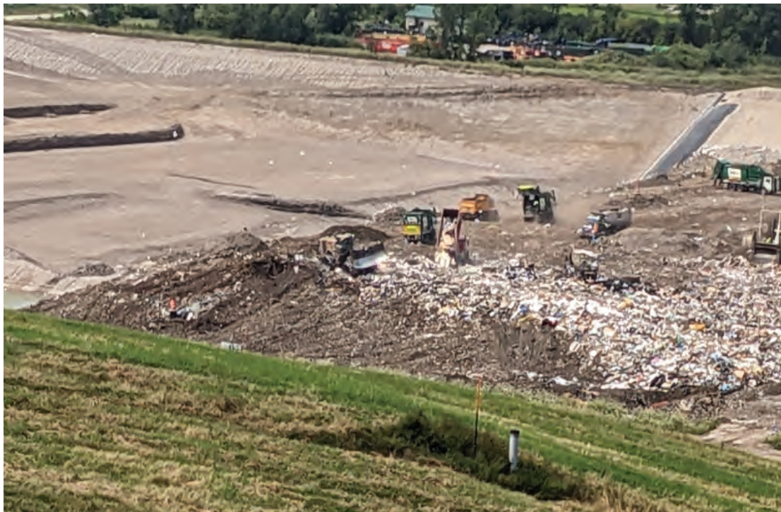
Dozer starting cover at Southwest corner of Phase 3
